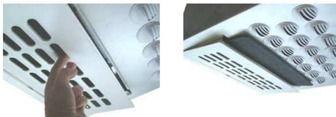
Insert a screwdriver, through an opening, into the hole in the clip, then incliner one of the lateral faces of the door towards the inside to disengage the retainer. Remove the door by pivoting it to disengage the retainer on the opposite side.
