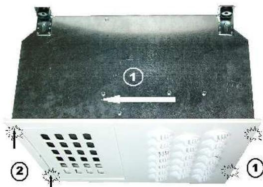
Raise the diffuser towards the unit, the locating lugs should clip to the diffuser, two clicks should be heard (2), the diffuser can now support itself.
